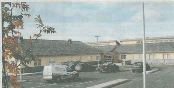
DEVELOPMENT: A new medical centre, similar to the one in Nefyn, will be built in Felinheli
